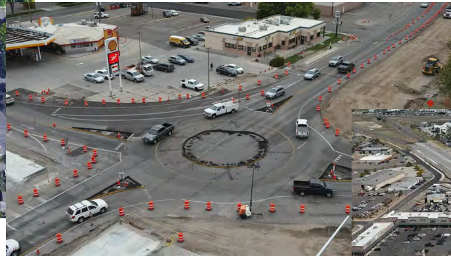
Temporary traffic circle
